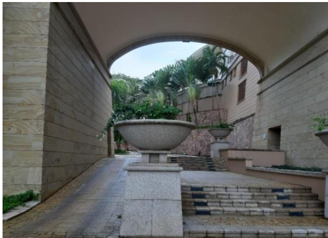
Ramps to access to hotel rooms (Pic: Tourism Development Department, Brunei)
