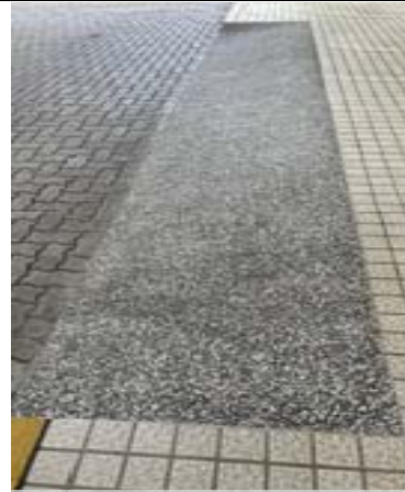
- WHEELCHAIR RAMP AT HOTEL MAIN ENTRANCE
