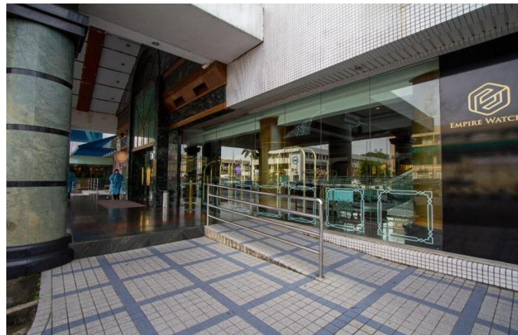
Ramp at the main entrance for access (Pic: Tourism Development Department, Brunei)
